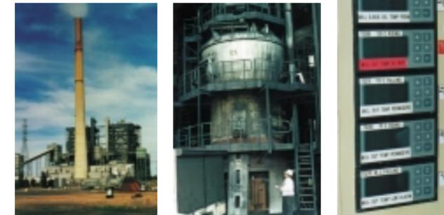
Coal used in power generation needs to be milled into a combustible state. It is an environment of dust, heat and vibration. Measurements on a mill are made primarily through a number of thermocouples directly connected to banks of UNIMETER XQLs. This information is linearized and calibrated to provide the correct sequence of switched outputs, which in turn controls the mill.
